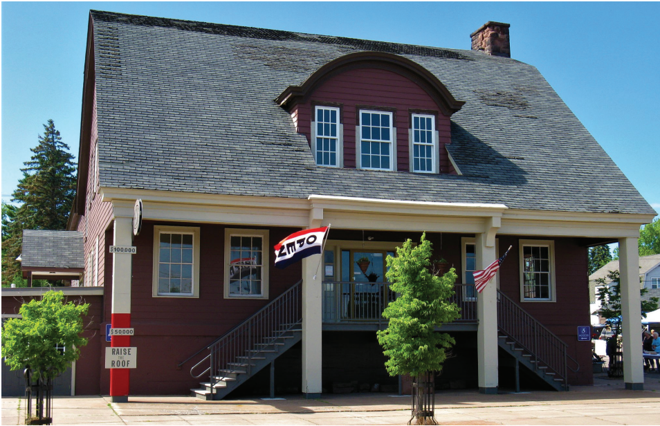
The Club is open for activities as renovation is restoring it to its original beauty.
